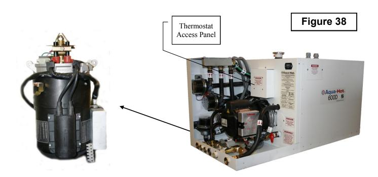
2. Carefully pull the Diesel-Burner away from the Aqua-Hot 4 to 5 inches before rotating the burner, and then remove.
