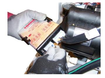
1. Locate the Diesel-Burner's Controller and disconnect both plugs. Failure to do so may result in the Diesel burner igniting.
