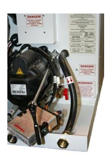
The Diesel-Burner is secured to the Aqua-Hot with two Eye Bolt Nuts that can be loosened, and swung out of the way by using a 10mm socket wrench with a 10 inch long extension.
