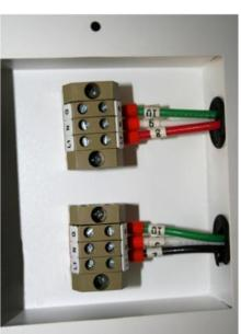
The Electric Element by disconnecting the wires NOTE: Test both the Hi-Limit Thermostat and And performing a Continuity Test.
