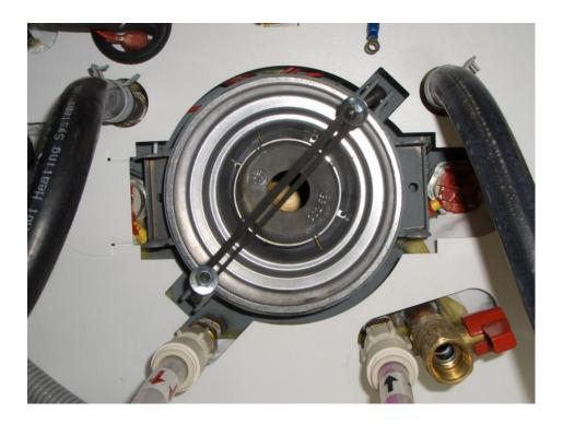
1. Reinstall the Combustion Chamber into the Aqua-Hot. Be sure to install the combustion chamber Seam in the 12:00 position. Failure to do so, may cause a crack to appear along the seam.
