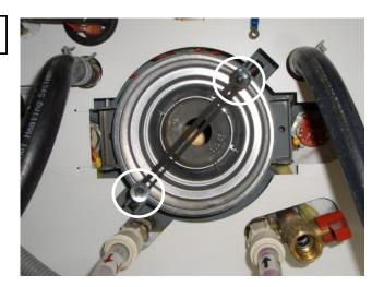
1. The Diesel-Burner is secured to the Aqua-Hot with two eye-bolt nuts that can be swung into place, after the diesel burner has been properly aligned and set in place.
